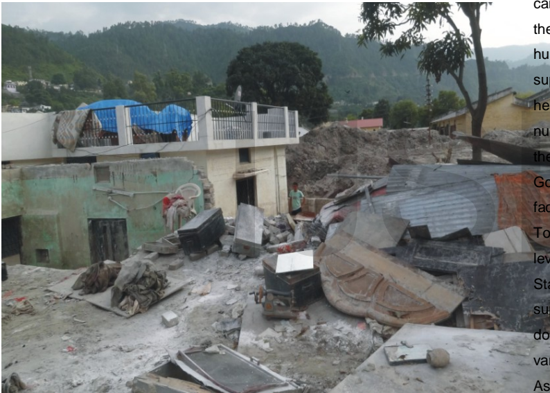
Photo 4: Residential buildings damaged due 16-17 June, 2013 flood disaster in Srinagar
