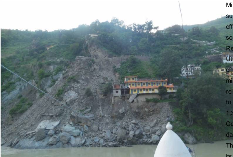
Photo 3: Many houses damaged due to landslide in Devprayag, Uttarakhand
